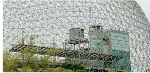
R. Buckminster Fuller’s geodesic dome created an innovative approach to enclosing space efficiently without supporting columns.
